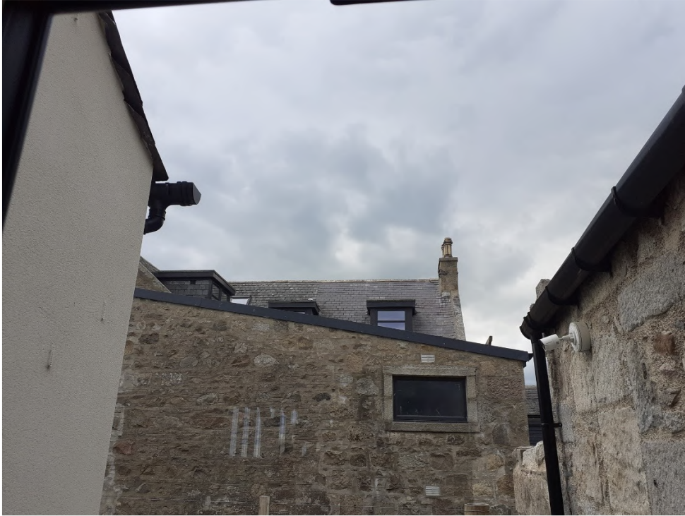
PHOTOGRAPH SHOWING VIEW of CRANFIELD GARAGE FROM 6 CRANFIELD STEADING – LINK
