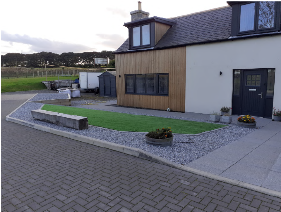
Existing Site Photograph
