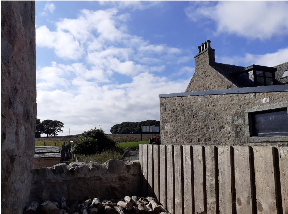
PHOTOGRAPH SHOWING VIEW of CRANFIELD GARAGE FROM ROAD OUTSIDE 6 CRANFIELD STEADING
