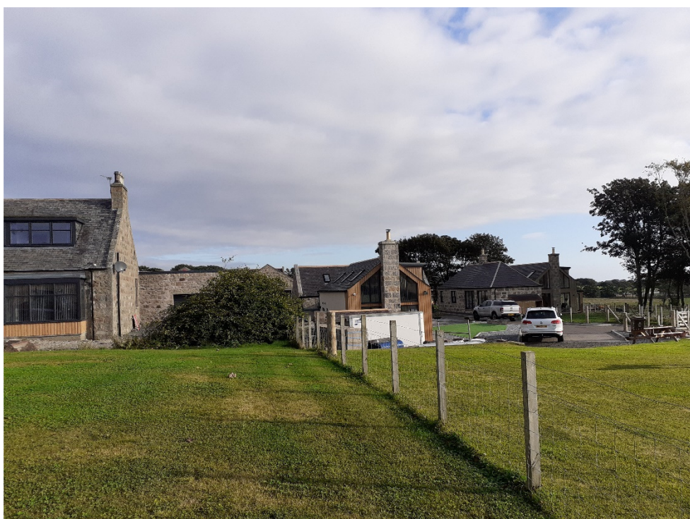
VIEW LOOKING AT 6 CRANFIELD STEADING FROM GARDEN OF CRANFIELD FARMHOUSE
